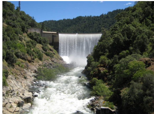
Slab Creek Dam
