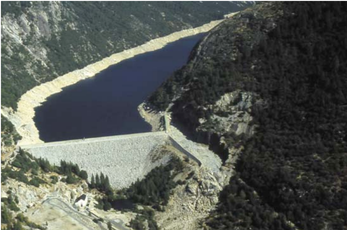
Salt Springs Dam on North Fork Mokelumne River
