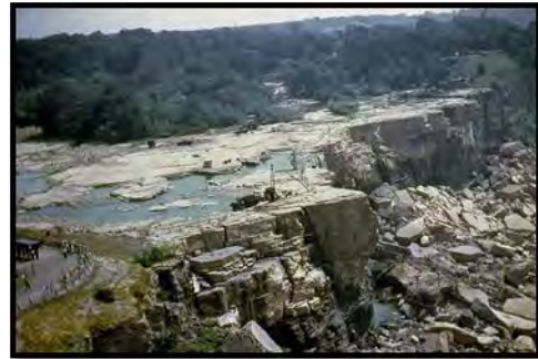
Engineers dried up the American Falls in 1969 to study erosion rates. Photo by Edwin H Schroeder.
