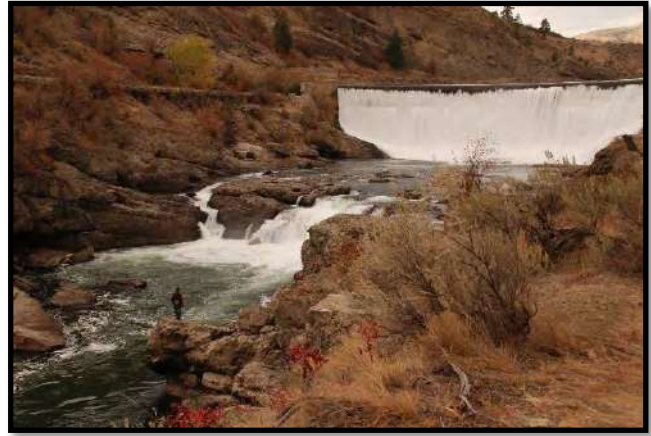
The Similkameen River flows over a 54 foot dam and 20 foot natural falls at about 700 cfs. A proposed hydro project would reduce flows to 10 to 30 cfs.
