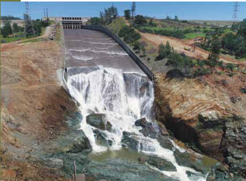
Main Spillway Erosion: A view of the erosion cavity at the Oroville main spillway – an infrastructural failure combining design, construction and maintenance issues. May 1, 2017. Source: Mike Burns, DWR.
