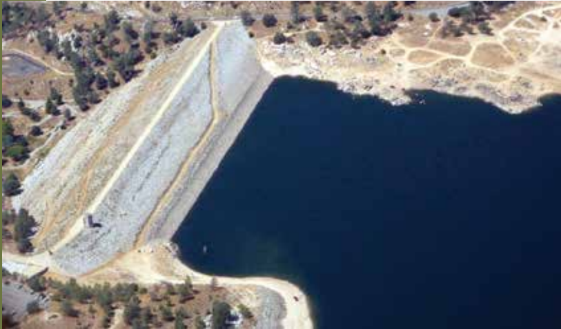
Isabella Dam on the Kern River gets a major seismic upgrade by the Army Corps of Engineers to reduce the risk of dam failure. Source: www.wikiwand.com/en/Isabella_Dam
