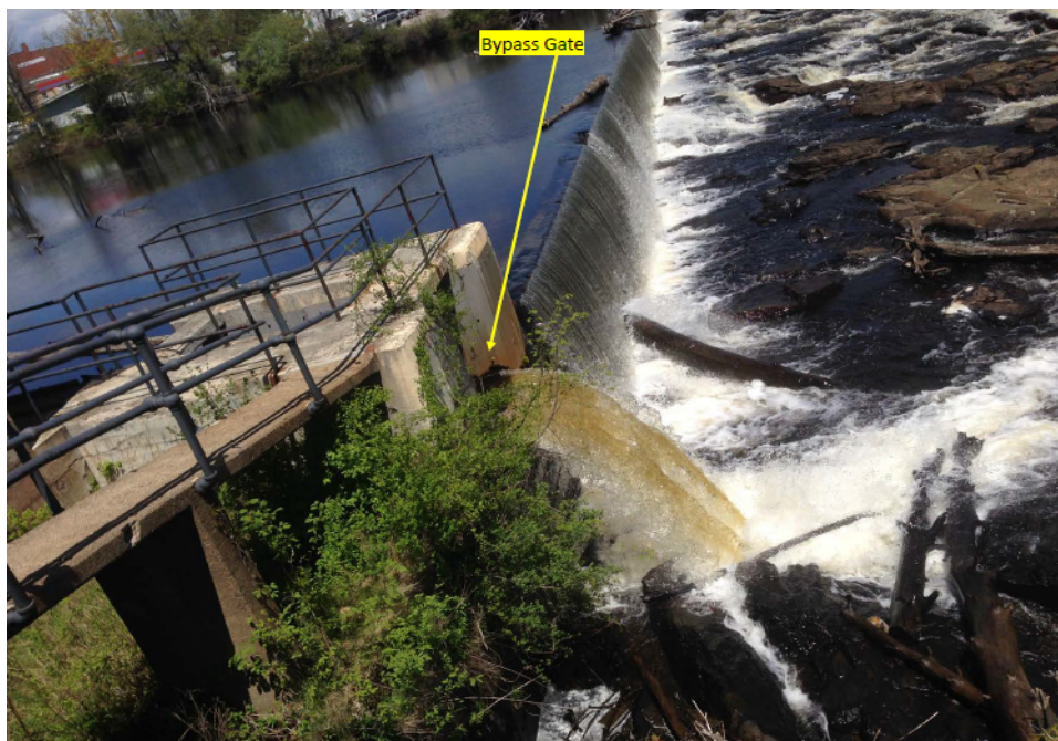
Photo 3: Stone Dam Bypass Gate shown in surrender application.
