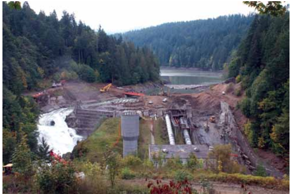
The Elwha Dam comes down in 2012. Photo by Thomas O'Keefe
