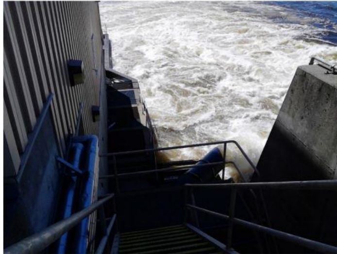
DOWNSTREAM FISHWAY PIPE AT THE WEST ENFIELD PROJECT
