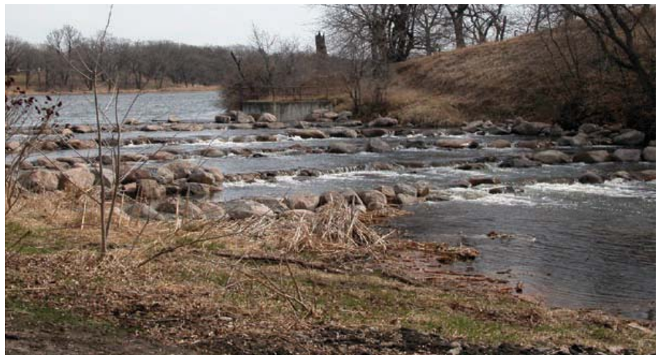
above: Lyons Park Dam rock ramp, Otter Tail River
